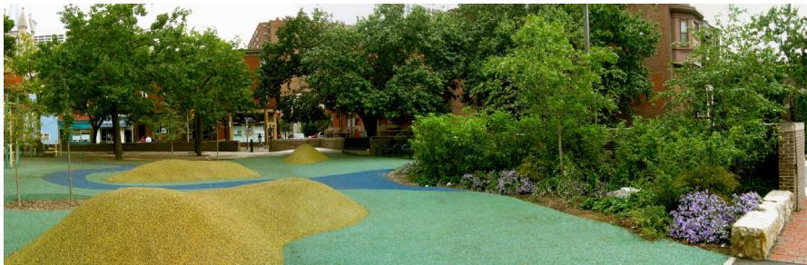
Phase 2 Rubber Surface Mounds and Bioswale Stormwater Plant Bed.
