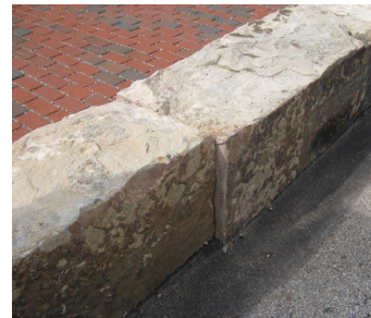
Recycled Bridge Abutments for Seating
