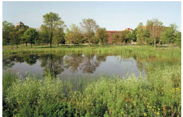
Constructed wetlands at the Immaculate Heart of Mary treat graywater from the facility
