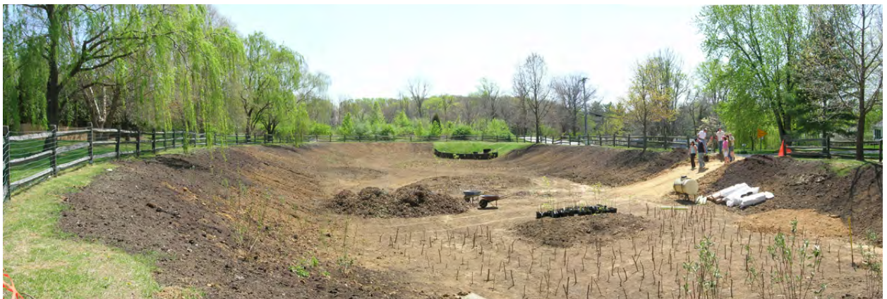
Live stakes (foreground) are simple to install and provide an inexpensive way to provide rapid shrub cover in the basin. Once established, the stakes will also provide structural reinforcement at the inlet, preventing the loss of soil during high-velocity flows.
